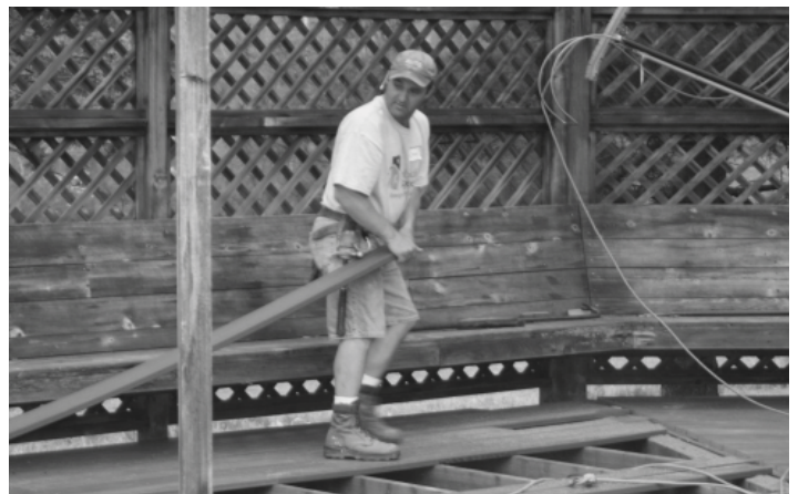
House captain Chris Giarrantano installs Trex decking at the Camp Friendship campgrounds in Laytonsville.
